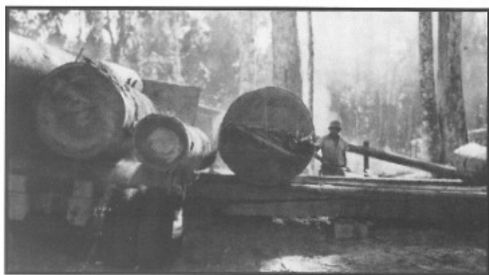
Typical load of logs
